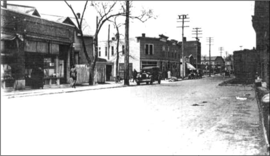
North on West Railroad (Greenbay) at Emerson (1924)
